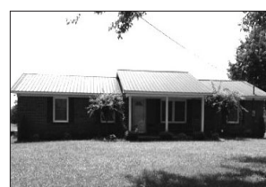
452 Lance Road 3 bedroom, 1 bath brick home
