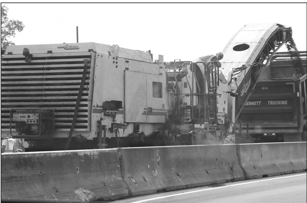
Work continues on the new four-lane extension of U.S. 70S between Woodbury and McMinnville, Due to recent problems completion has been rescheduled until November. MIKE WEST photo
