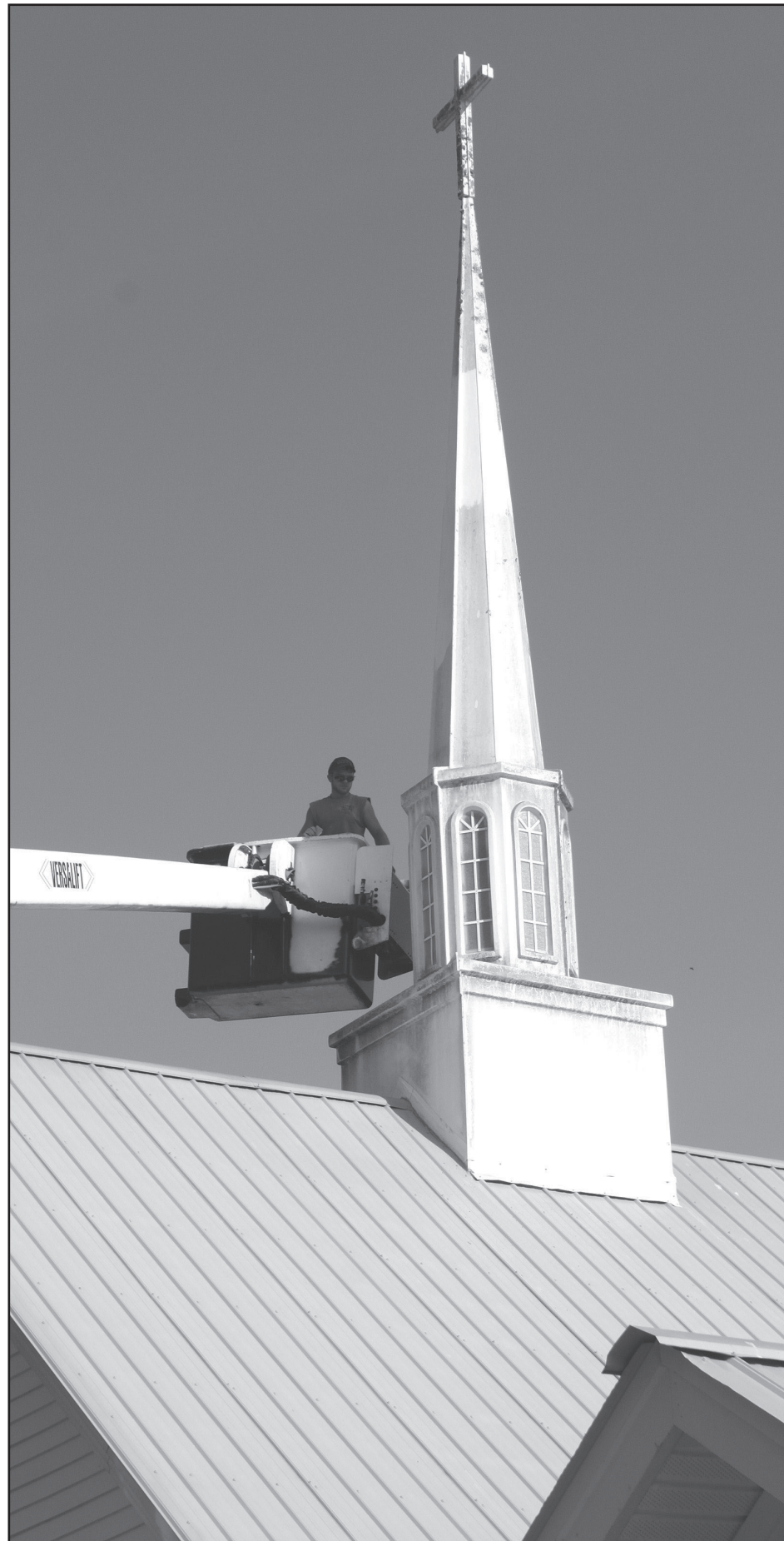
MIKE WEST photo David Goff prepares the steeple of First United Methodist Church for painting. David, who works with Goff Tree Services, then painted the steeple with paint designed to last at least 10 years..
