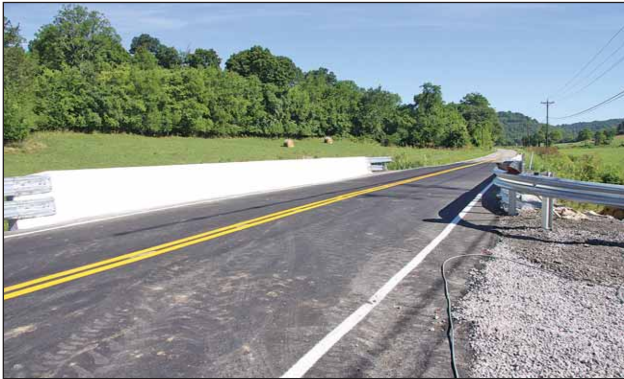
It's smooth sailing once again on state Route 145 between Woodbury and Auburntown. A new bridge over Rush Creek was completed in record time ... 21 days ... replacing the old bridge of undetermined age. See Page 12 for more photos.
