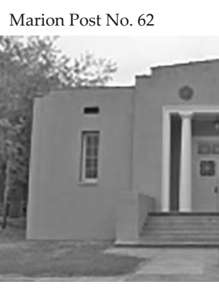
The American Legion Clubhouse, historically known as Marion Post No. 62, is located at 300 Elm Avenue, South Pittsburg, Marion County and was nominated to the National Register for its local significance in architecture and social history.
