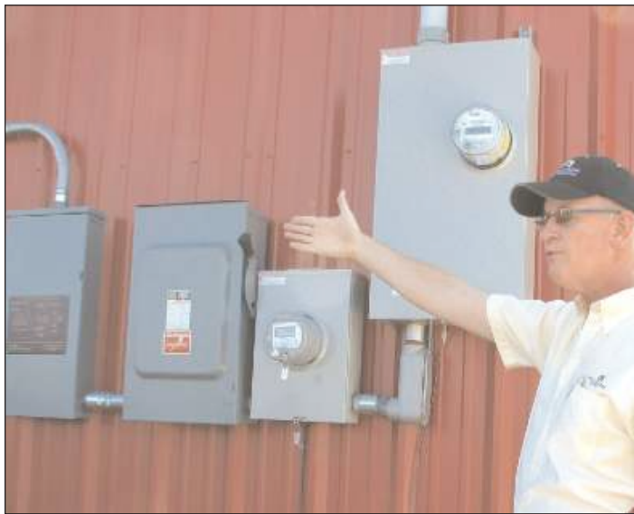
John Barker with Middle TN Electric Membership Corporation explains the solar grid tie interconnection during the recent solar tour at the Cannon County Arts Center.
