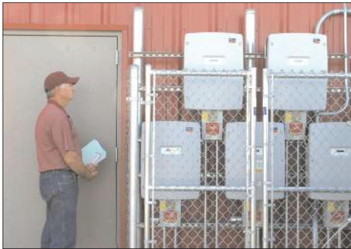
A tour visitor assessing the power inverters.
