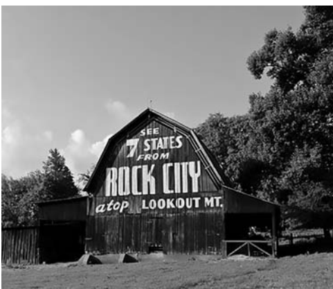
The "before" shot prior to the repaint - this barn was built 90 years ago (1926)
